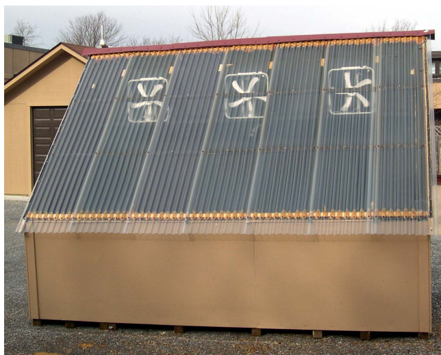
Figure 5. Front view of kiln showing fan placement.
