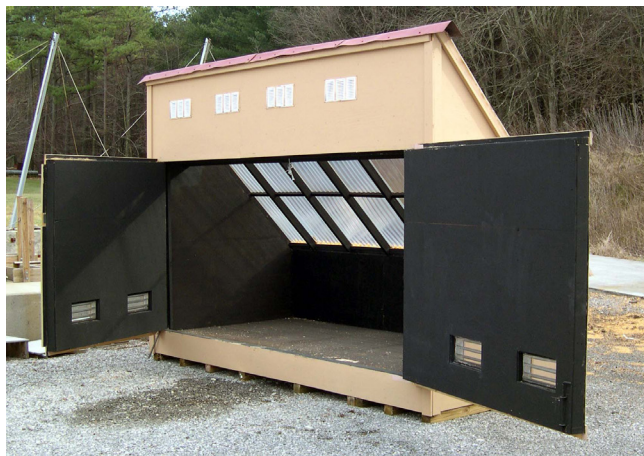
Figure 4. Rear view of kiln showing access doors.
